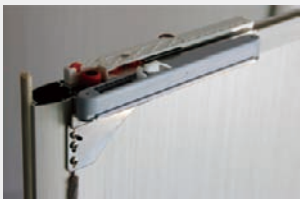
The lower locator is installed on the back of the mullion
