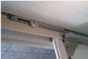
The upper locator is installed on the back of the upper track
