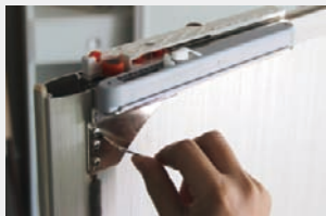
Adjust the parallelism with the sliding door plane
